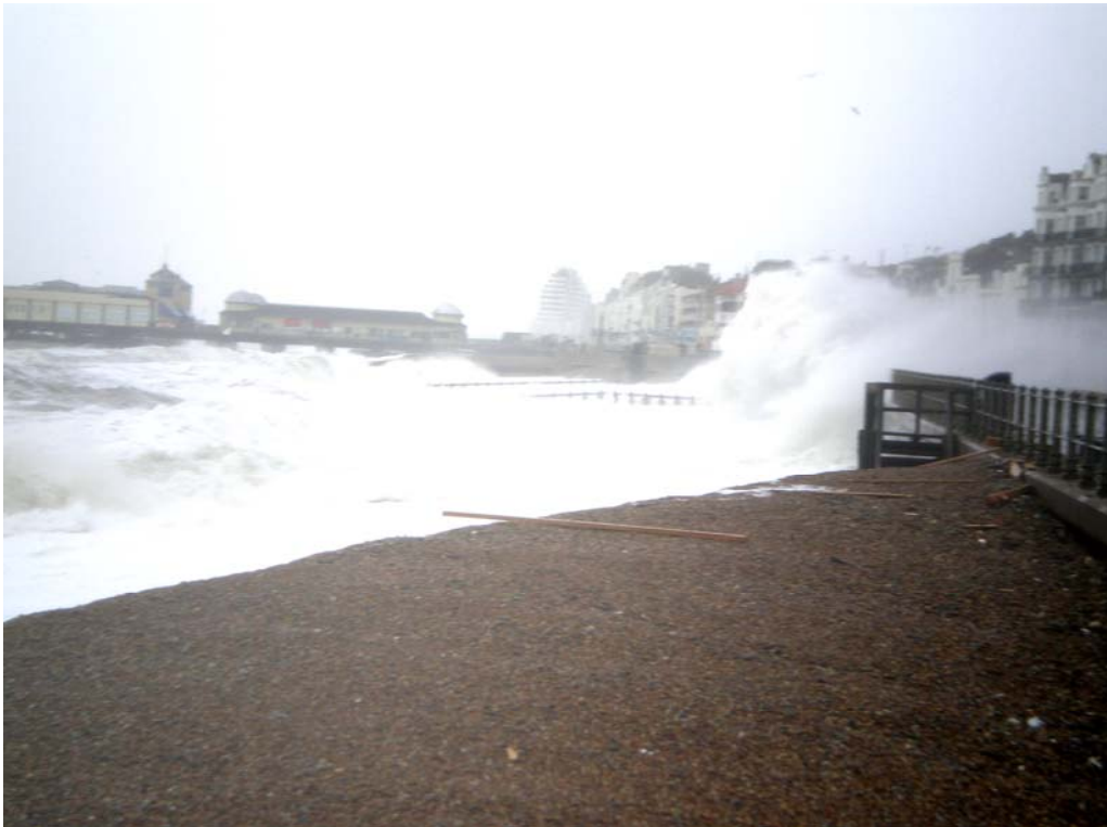
Figure 3.1: Impact of a Recent Storm Event at Hastings Prior to Remedial Works in 2009
