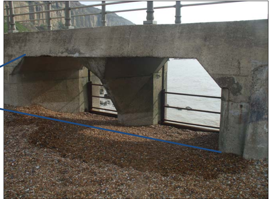
Figure 5.2: Open Sluice Gate inside the Harbour Beach
