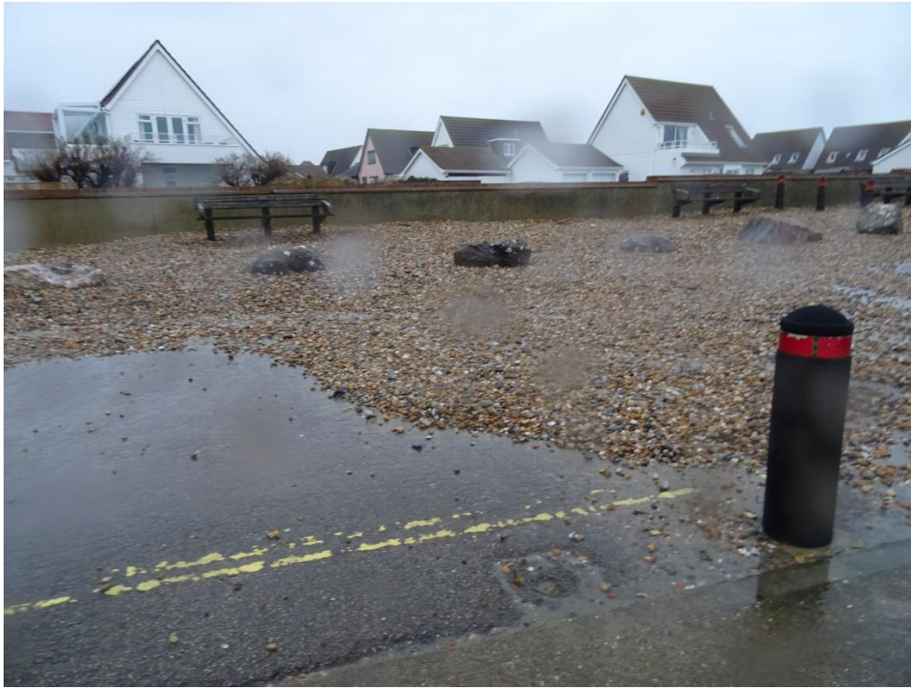
FIGURE 6-2-8 EVIDENCE OF OVERTOPPING ON TO THE PROMENADE, SELSEY (2016)
