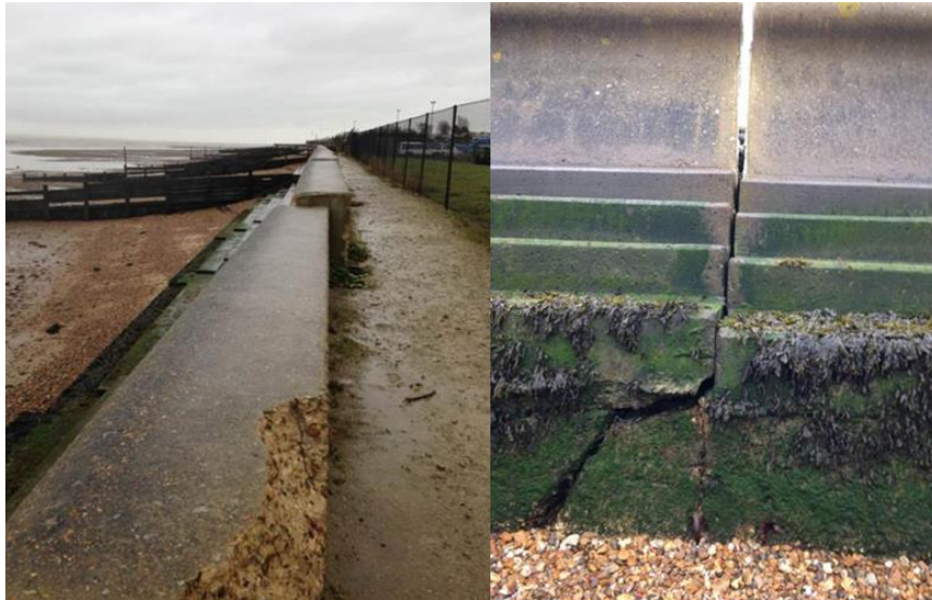
FIGURE 6-2-13 FAILURE OF A SEAWALL AT ALL HALLOWS DUE TO SLIDING/TOPPLING OF DEFENCE SECTIONS (2015)
