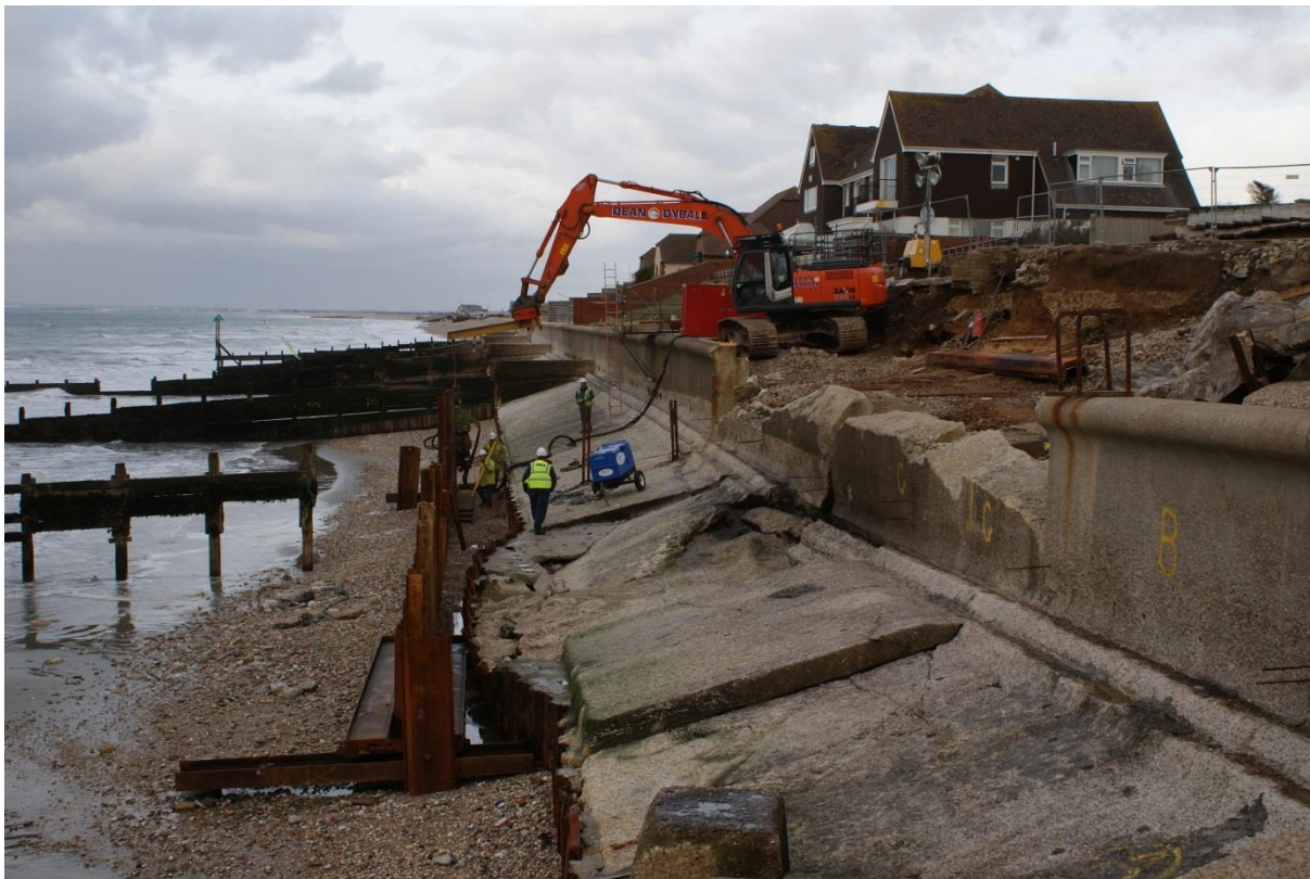
FIGURE 6-2-11 DILAPIDATED GROYNES, LOW BEACH AND SEAWALL FAILURE AT SELSEY (2008)
