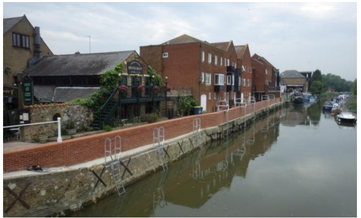
Right: Aynsley Court, Sandwich: After our tidal defence works.
