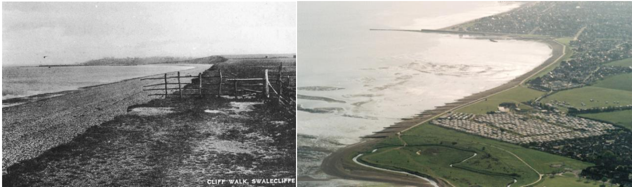
Figure 4-18 Swalecliffe prior to the construction of a seawall (probably pre-1900) and in 2010
