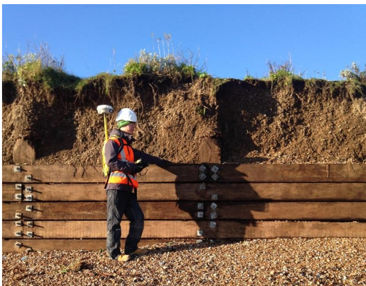
FIGURE 8-1 EXPOSED TIMBER BREASTWORK AND CLIFFING AT WELLINGTON PARADE (JAN 2016)
