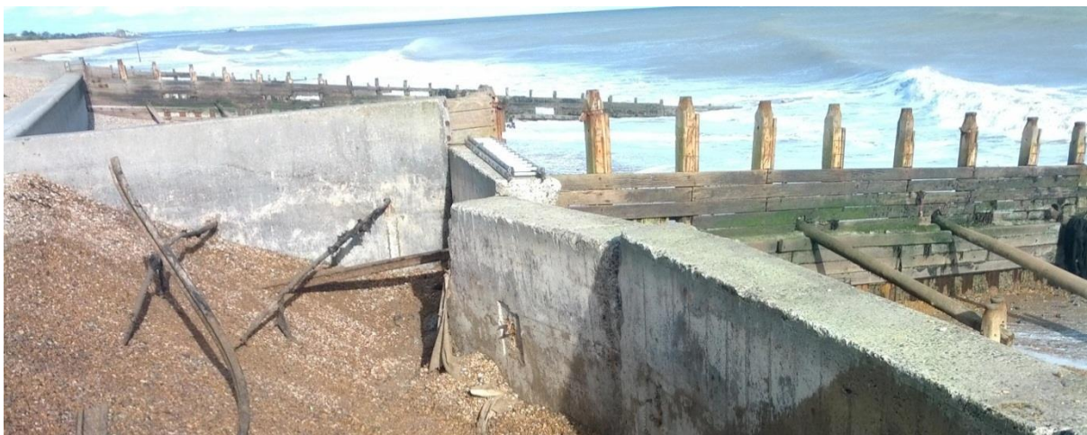
FIGURE 6-2-11 DILAPIDATED GROYNES, LOW BEACH AND SEAWALL FAILURE AT KINGSDOWN (2013)
