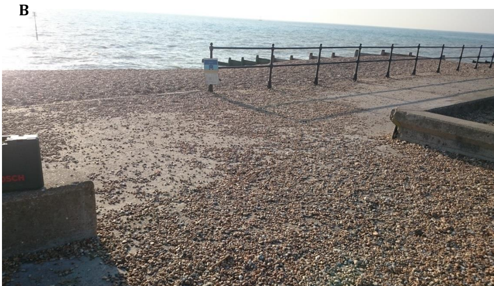
FIGURE 6-2-8 EVIDENCE OF OVERTOPPING IN DEAL (A) ON THE PROMENADE IN CENTRAL DEAL AND (B) AT KINGSDOWN (BOTH PHOTOS 2016)
