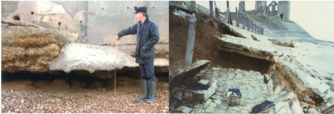
FIGURE 6-2-12 EXAMPLES OF UNDERMINING AT TANKERTON (LEFT) AND RECVLVER (RIGHT) (BOTH PHOTOS 1999)
