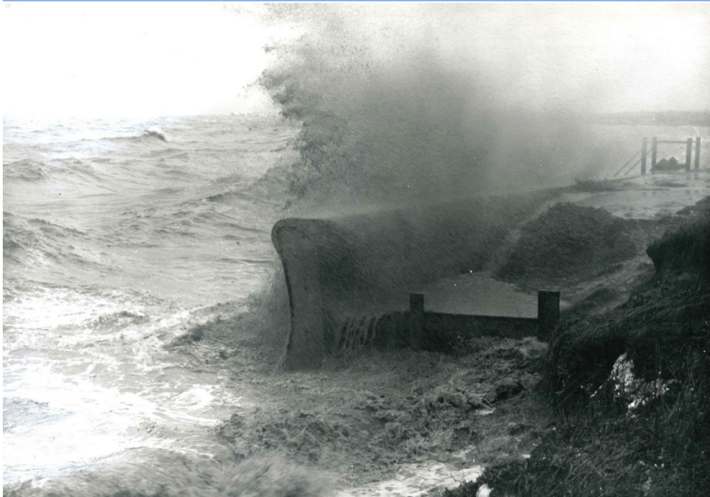
FIGURE 6-2-8 OVERTOPPING AT SWALECLIFFE, 1953
