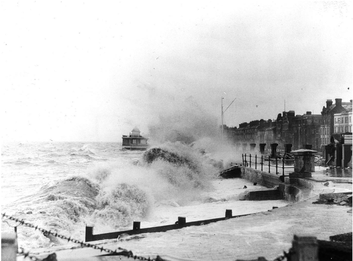
FIGURE 6-2-11 OVERTOPPING AT HERNE BAY, 1953
