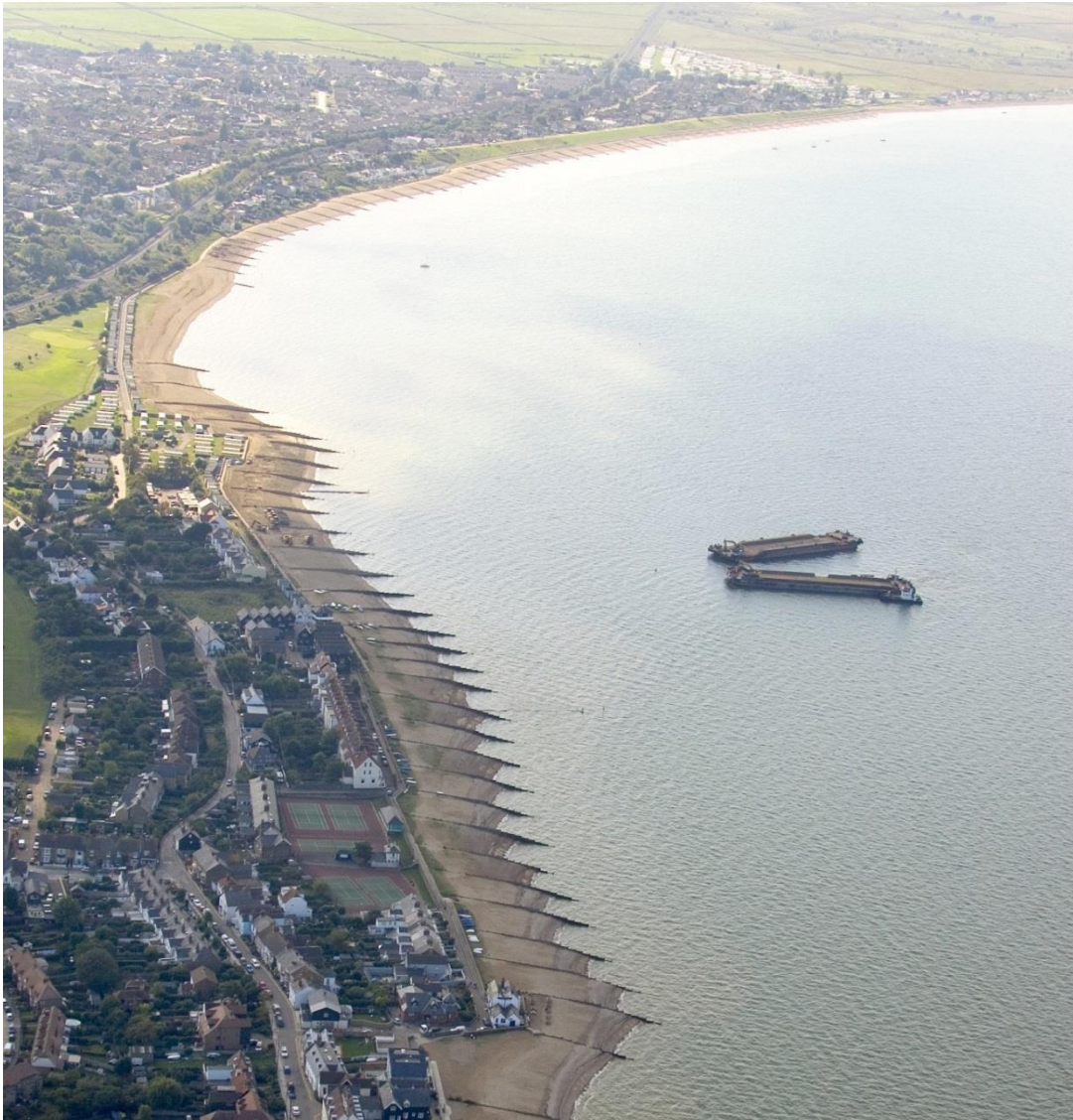
FIGURE 1-10 NEW TIMBER GROYNES AND BEACH REPLENISHMENT: THE 2006 CAPITAL SCHEME
