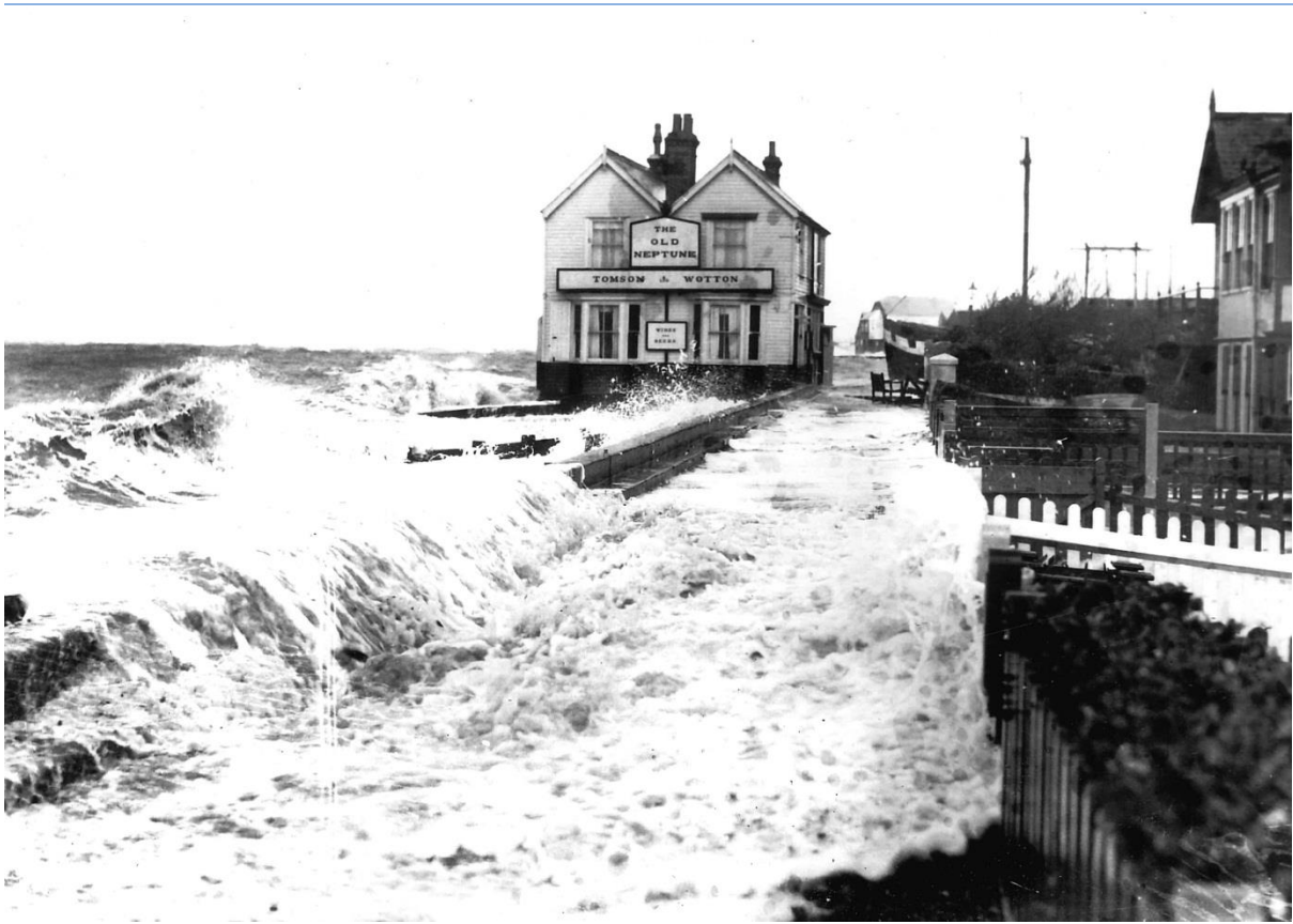
FIGURE 6-2-10 OVERTOPPING AT WHITSTABLE, 1978
