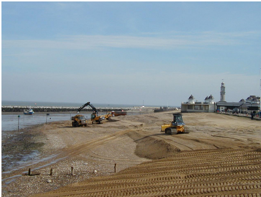
FIGURE 8-8 BEACH RECYCLING WITHIN THE HARBOUR SECTION H (EAST CLIFF PARADE)
