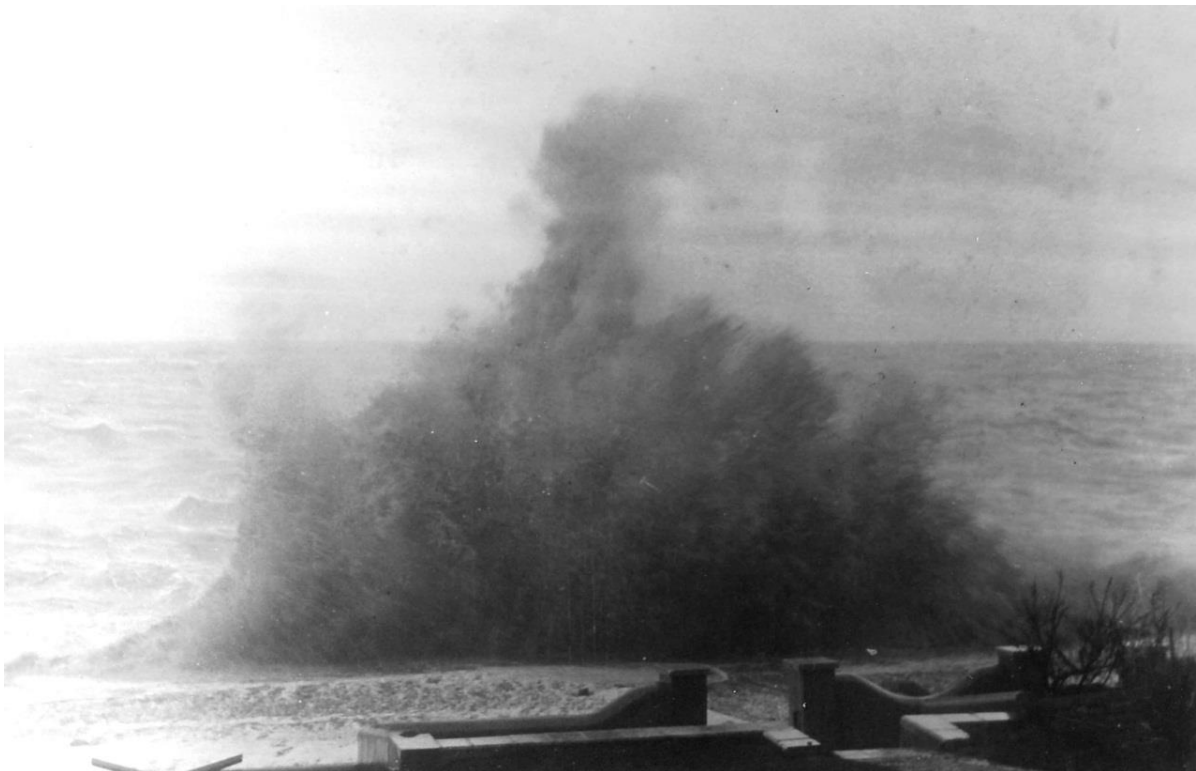
FIGURE 6-2-9 OVERTOPPING AT HERNE BAY, 1953
