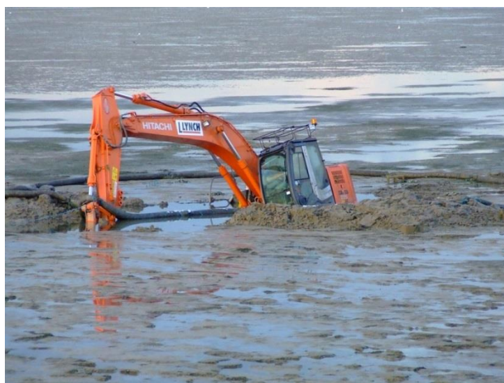
FIGURE 8-3 EXCAVATOR LOST IN THE DEEP MUD DURING THE WINDFARM CABLE INSTALLATION
