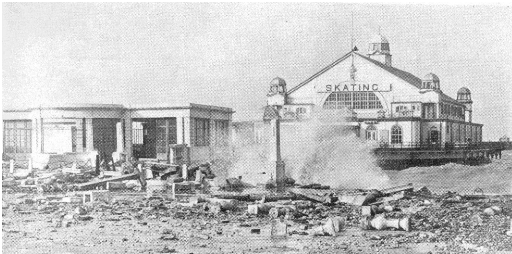
FIGURE 6-2-7 OVERTOPPING AT HERNE BAY PIER, 1953
