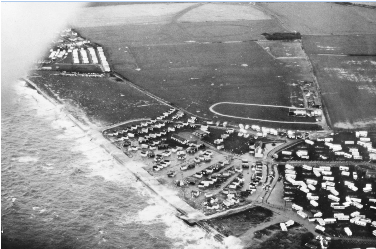
FIGURE 6-2-12 OVERTOPPING AT SWALECLIFFE, 1953
