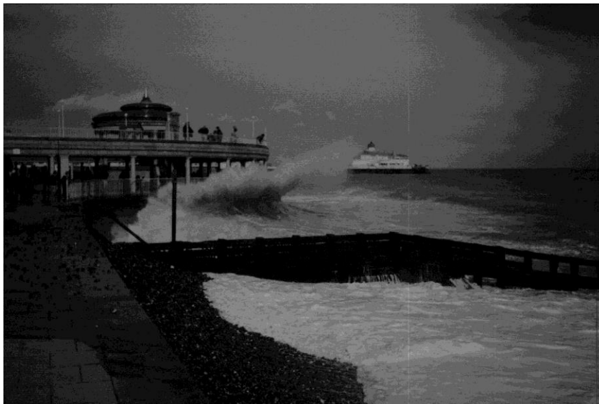
FIGURE 6-2-8 OVERTOPPING AT EASTBOURNE IN THE 1990S (BEACH LEVELS LOWER THAN PRESENT DAY)
