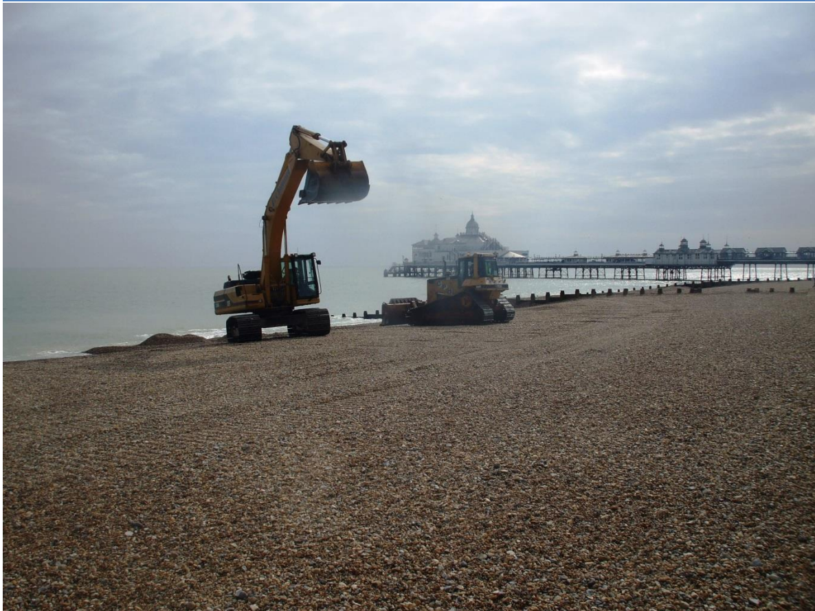
FIGURE 8-1 RECYCLING WORKS AT EASTBOURNE PIER, 2012
