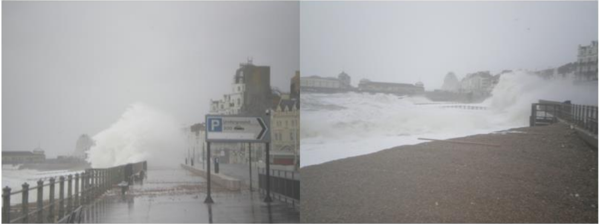
FIGURE 6-2-7 SEVERE OVERTOPPING AT HASTINGS AS A CONSEQUENCE OF LOW BEACH LEVELS (2009)
