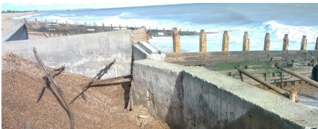
FIGURE 6-2-12 DILAPIDATED GROYNES LOW BEACH AND SEAWALL FAILURE AT KINGSDOWN
