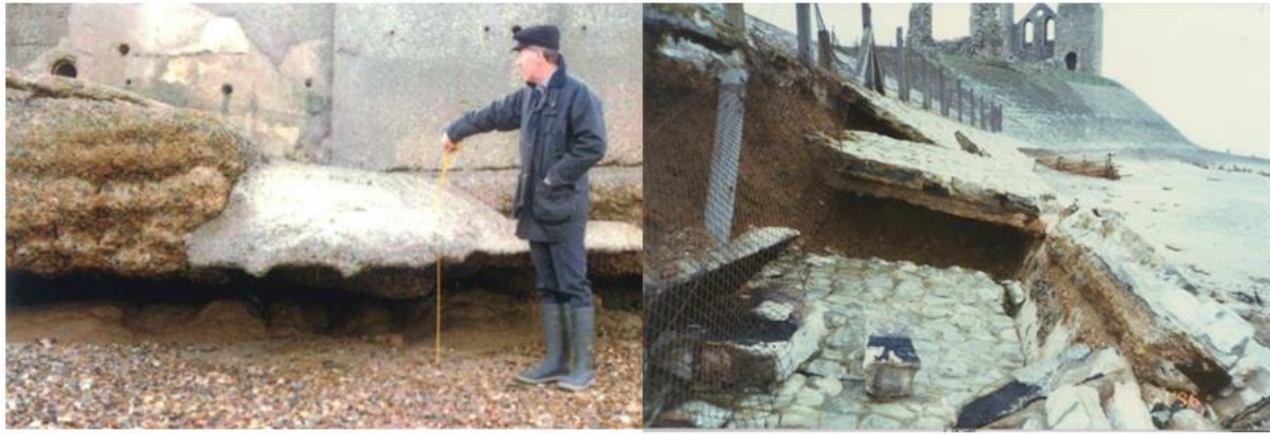
FIGURE 6-2-13 EXAMPLES OF UNDERMINING AT TANKERTON (LEFT) AND RECVLVER (RIGHT)
