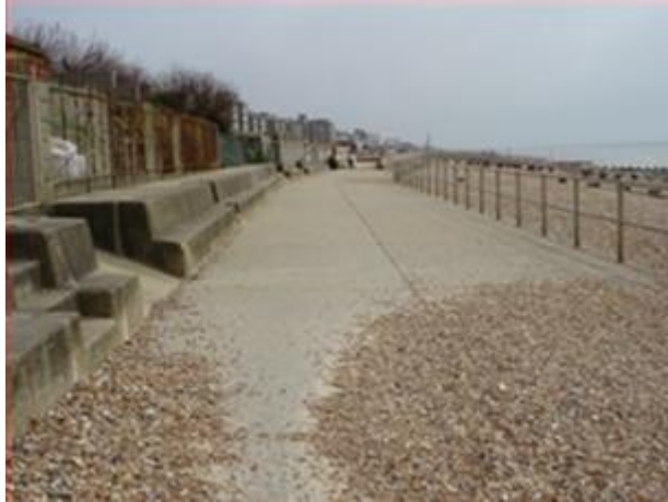
FIGURE 6-2-9 SHINGLE WASHED ON TO THE PROMENADE AT BEXHILL (2015)
