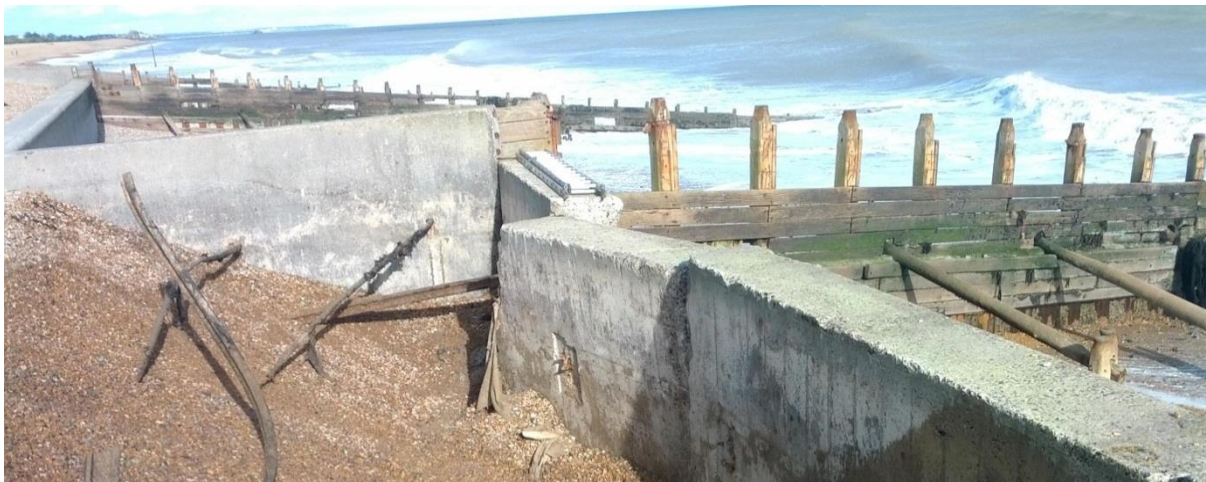
FIGURE 6-2-11 DILAPIDATED GROYNES, LOW BEACH AND SEAWALL FAILURE AT KINGSOWN (2013)
