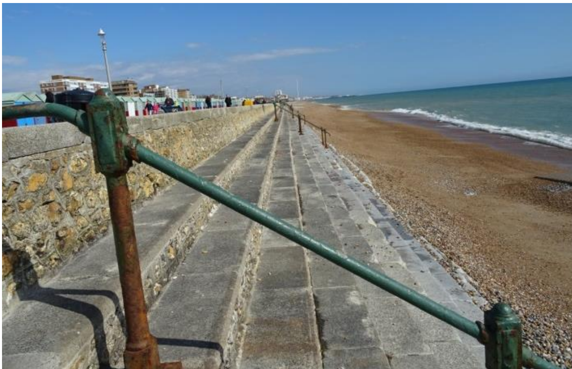
FIGURE 1-11- STEPPED REVETMENT, HOVE
