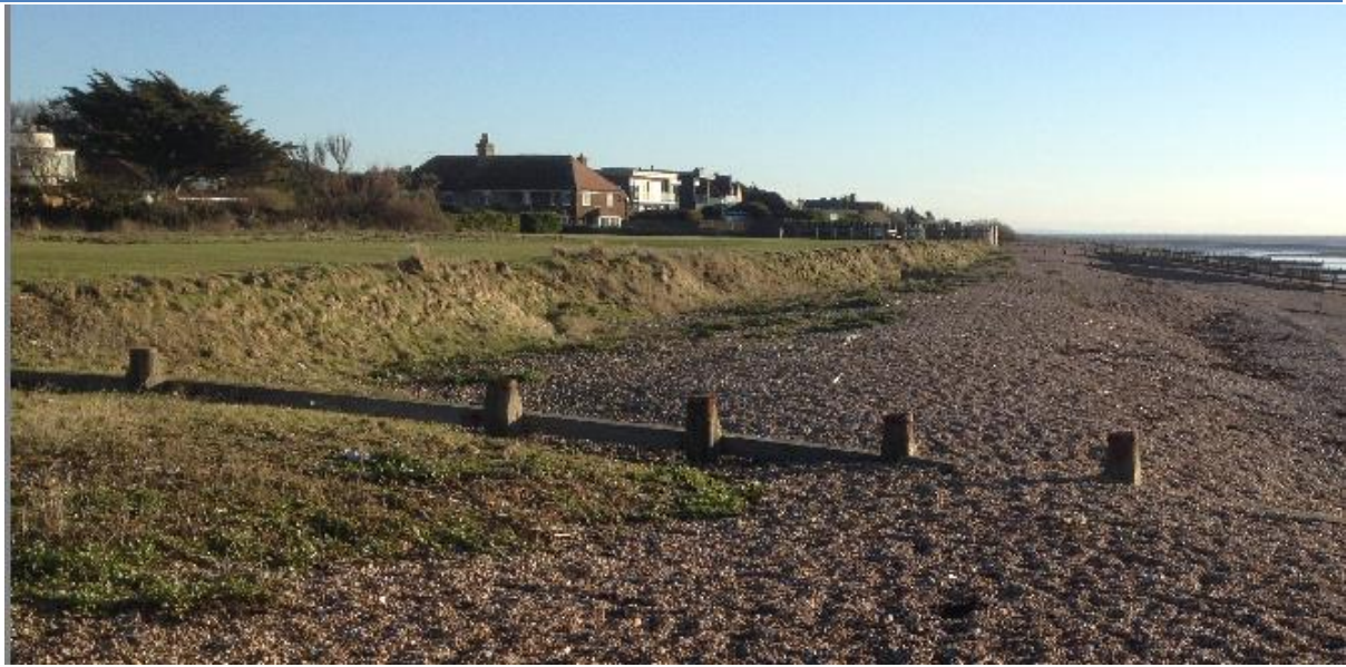
FIGURE 2-1 WOODEN GROYNES AND SHINGLE BEACH FRONTING RISING GROUND, LOOKING TOWARDS FERRING FROM RUSTINGTON
