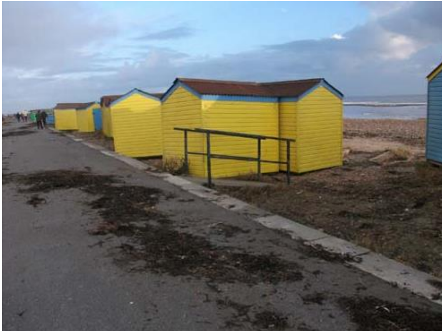
FIGURE 6-2-8 EVIDENCE OF OVERTOPPING ON TO THE PROMENADE, LITTLEHAMPTON (2014)
